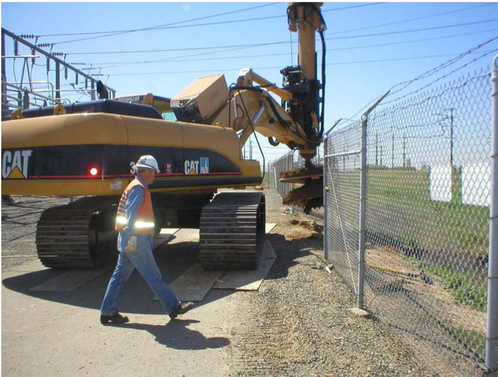
**Figure 4** – Crews drilling Pole #1 just outside the Atlantic substation on the west side. April 20, 2005.
