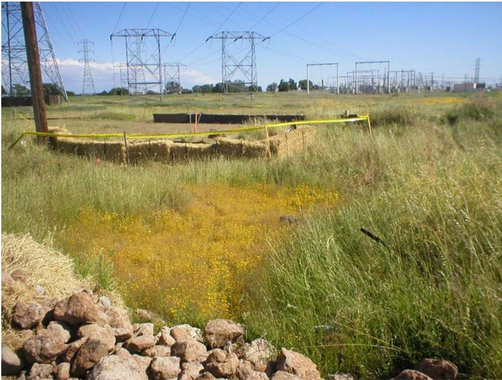
**Figure 3** – Vernal pool area (foreground) protected by installed erosion controls surrounding Pole #4. April 19, 2005.
