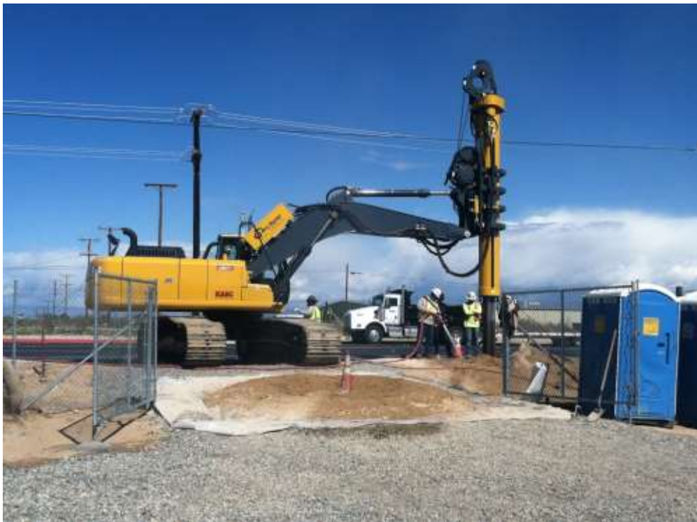
Figure 2 – Augering for TSP foundation occurred during the subject period. View northeast, 03/03/15.
