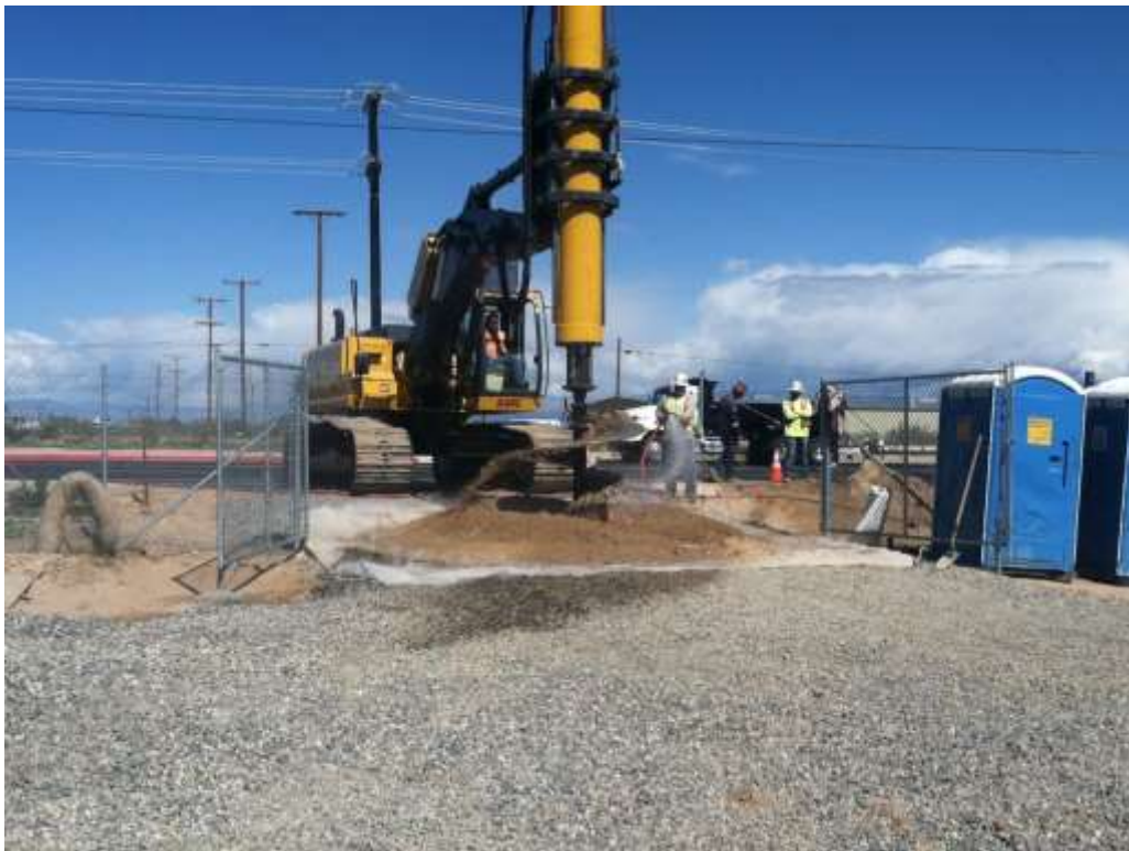
Figure 3 – Dust control measures were implemented during the subject period. View northeast, 03/03/15.
