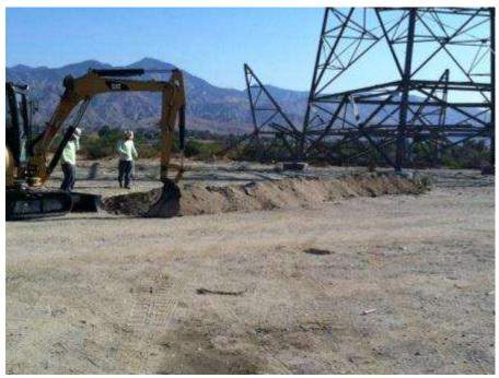
Figure 7. Trenching for grounding wire at Tower 1061.
