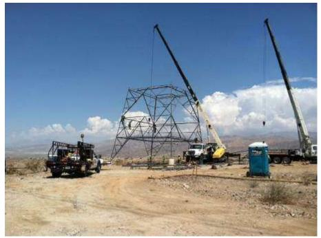
Figure 4. Tower erection activities at Tower 2250.
