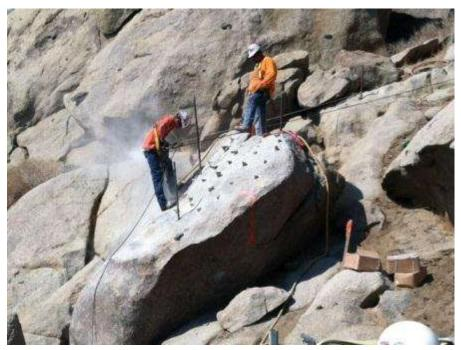
**Figure 6.** Rock clearing activities at Tower 1034. This rock is being prepared for the addition of Dexpan compound to break-up the rock.
