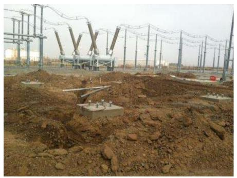
Figure 10. Trenching for the grounding wires for foundations within the Valley Substation.
