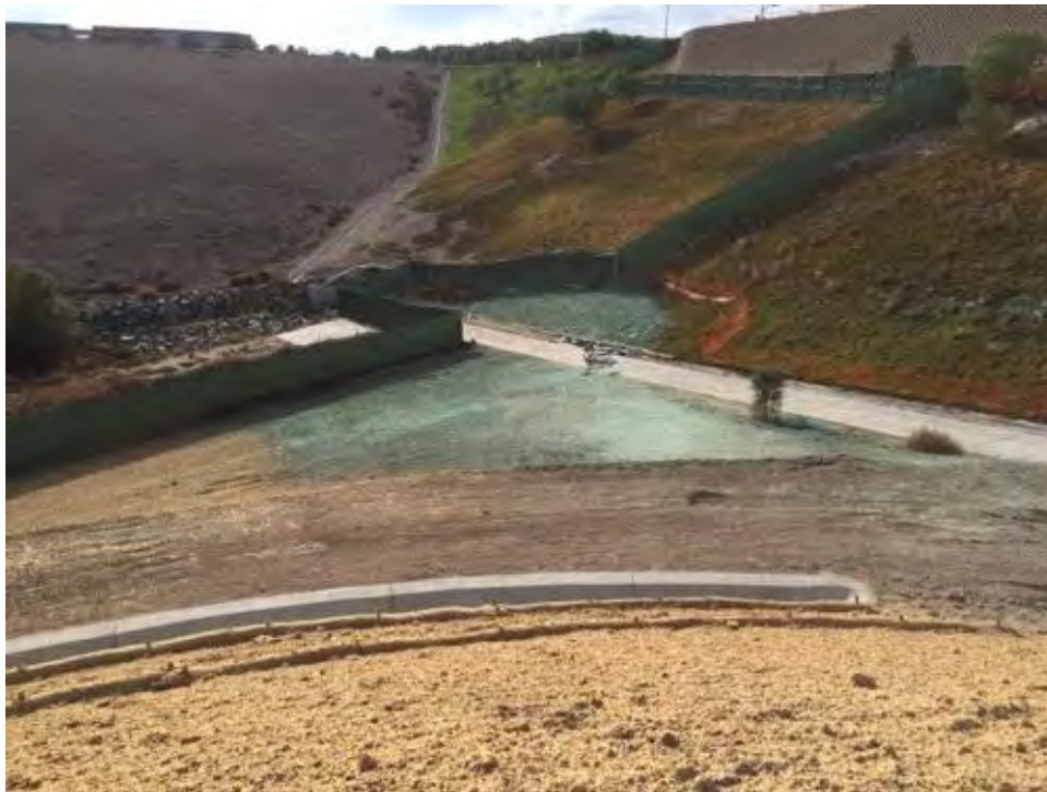
Caption Addition BFM sprayed on slope in northwest corner.
