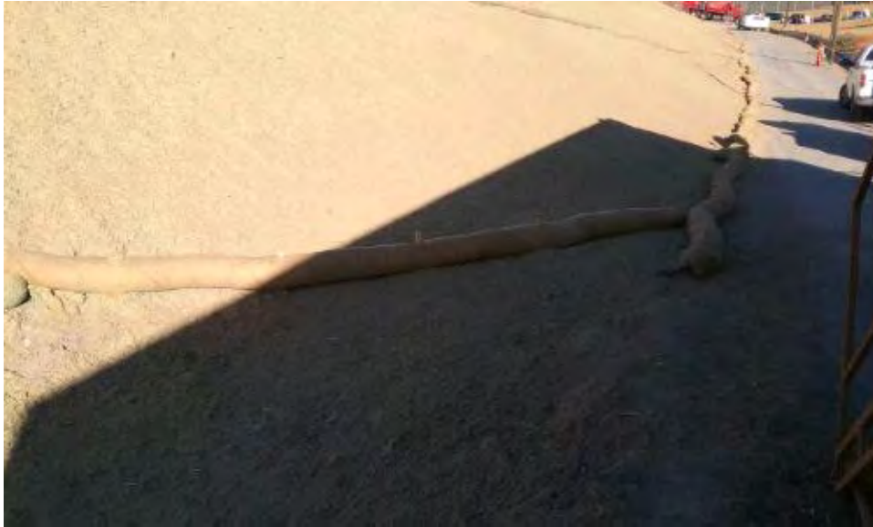
Caption Straw wattle in place near construction trailer.
