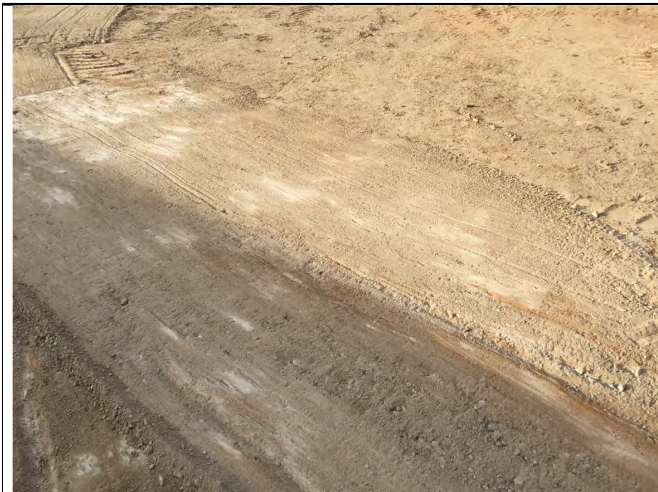
Photograph 4: Area where hydraulic fluid spill occurred after clean up on November 15, 2016.
