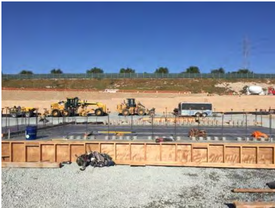
Caption Foundation for the control house
