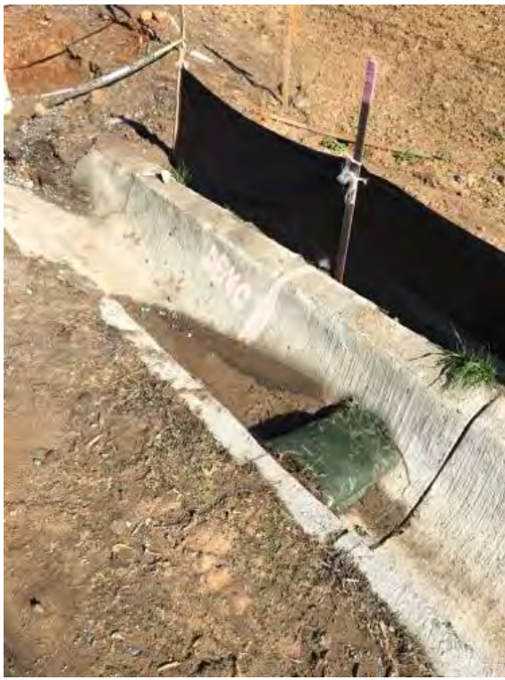
Caption Sediment trap in culvert
