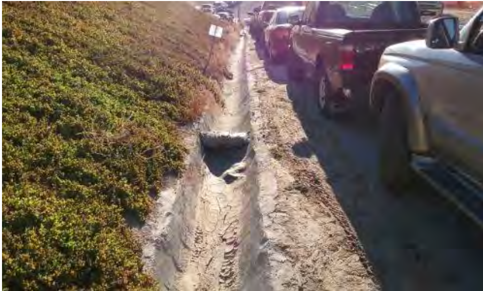
Caption Erosion control in eastern brow ditch functioning.
