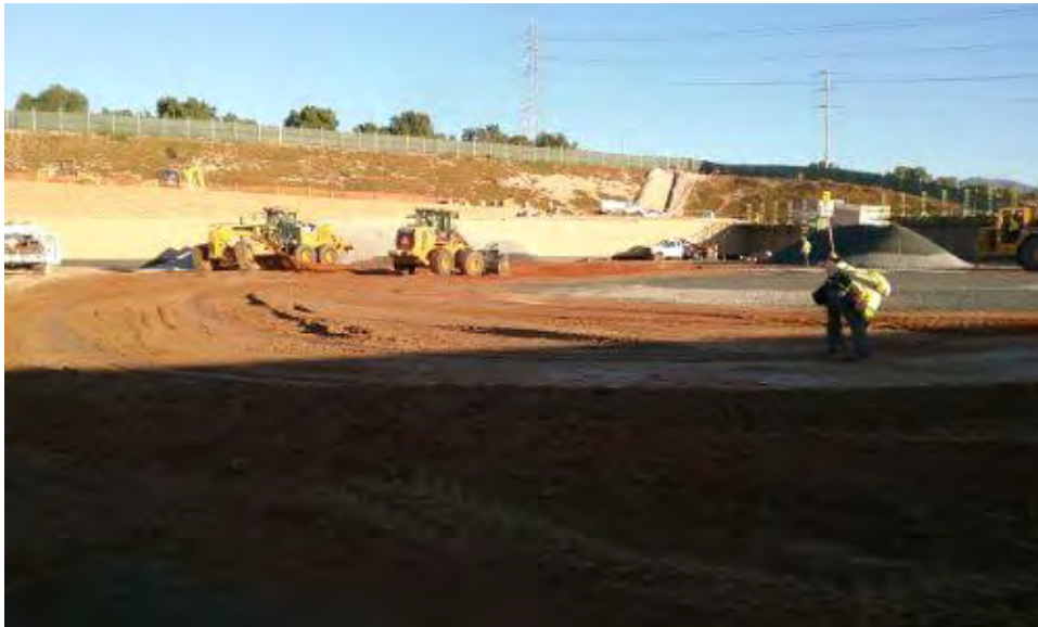
Caption Spreading and mixing fill for substation pad.
