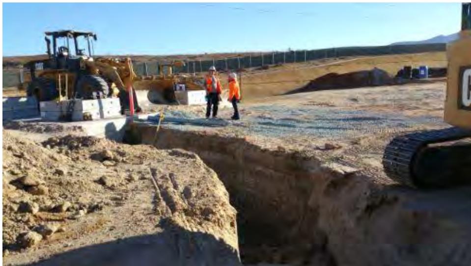
Caption Paleontological monitor observing excavation.
