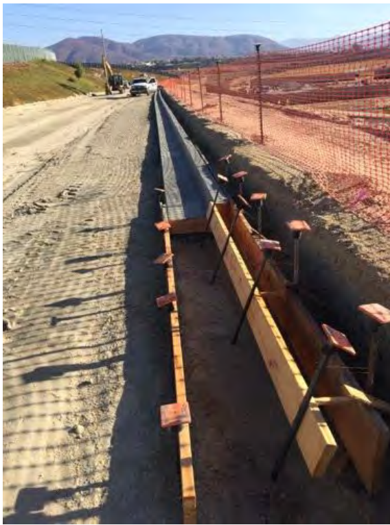
Caption New curb and gutter along Access Road A
