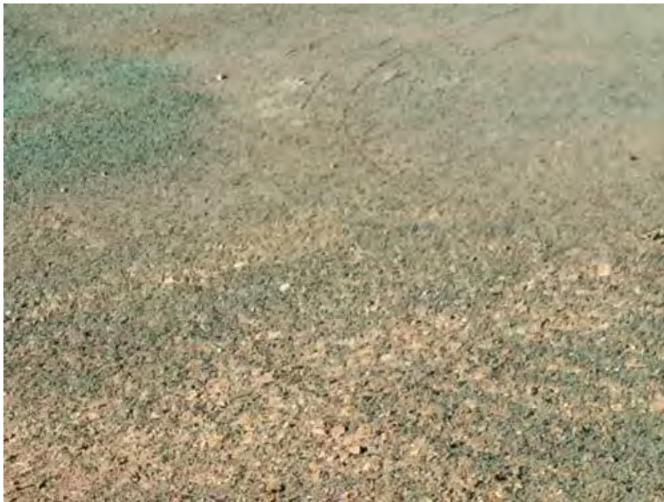
Caption BFM applied thinly on NW slope
