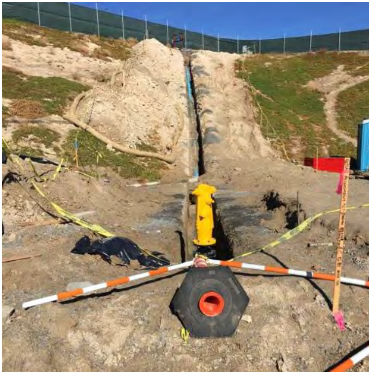
Caption Open trench
