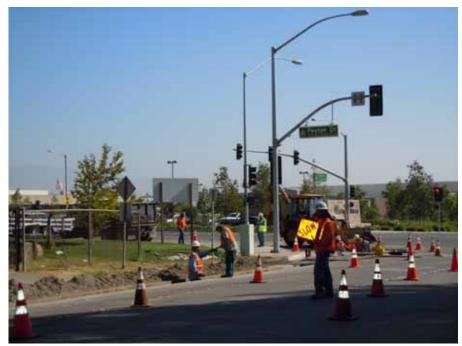
**Figure 5:** Segment 8 Telecom trenching work along Peyton Drive in Chino Hills.
