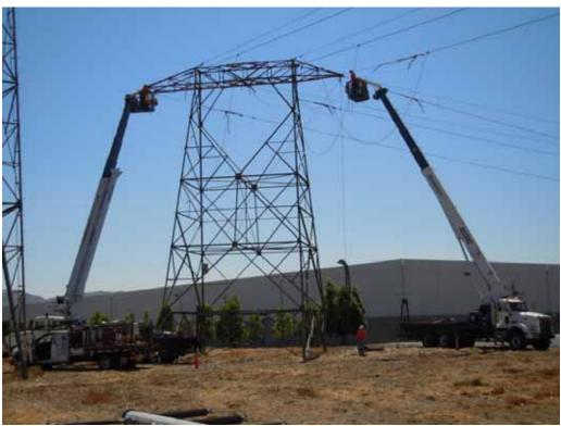
**Figure 6:** Segment 8 Phase 1 crews attach travellers to wreck-out towers in preparation to remove 220 kV wire.
