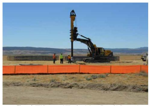
**Figure 2:** KV Structures drilling foundation at Tower 34, Segment 4.
