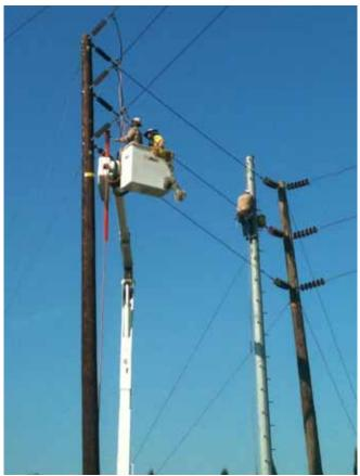
**Figure 4:** 66 kV crews working on the Rio Hondo-Amador-Jose-Mesa Line loosen wire on an old pole (left) and install cross-arms on a new pole in a nursery in Baldwin Park (right).
