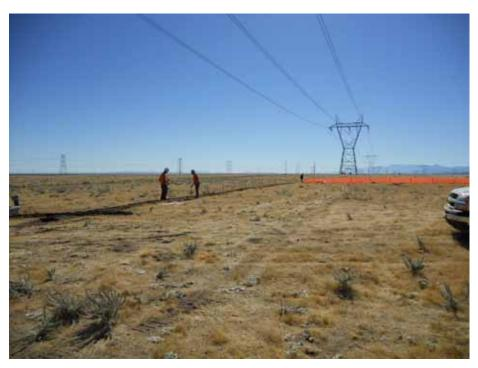
Figure 3: H&H Grading installing silt fence at Tower 34, Segment 4.
