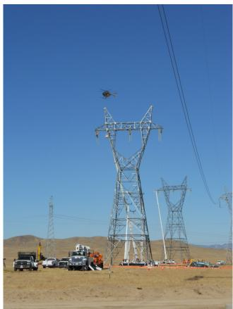
**Figure 1:** Segment 4, wire stringing at Towers 34 & 35 for the LADWP crossing.
