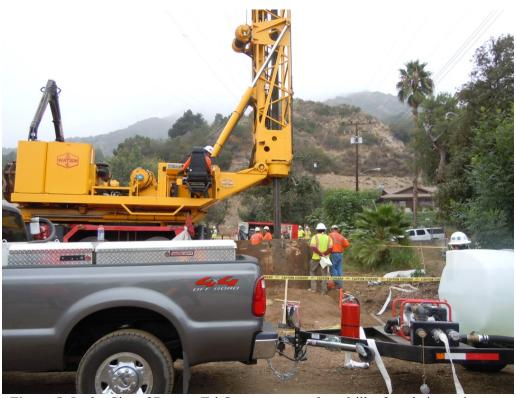
**Figure 5:** In the City of Duarte, Tri-State crews work to drill a foundation at interset tower M54-T3a on Segment 7.
