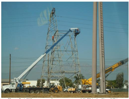
**Figure 3:** A Wilson crew works to remove tower M0-T3 in the City of Chino, Segment 8 Phase 2.
