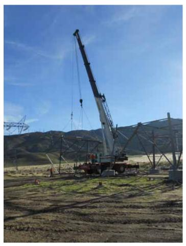
**Figure 1:** Steel crew assembling 500 kV Tower 38, Segment 5.
