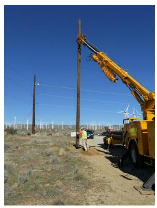
**Figure 3:** H&M pole setting crew at intersection of Oak Creek Road and 90<sup>th</sup> Street, Segment 10 Telecom.
