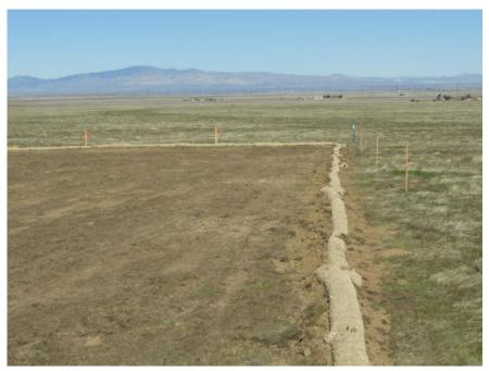
**Figure 1:** Site preparation and fiber roll installation at project disturbance areas, Segment 4.
