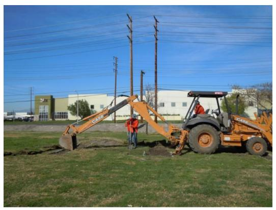
Figure 7: Crews work on installing an artificial owl burrow in the City of Chino.
