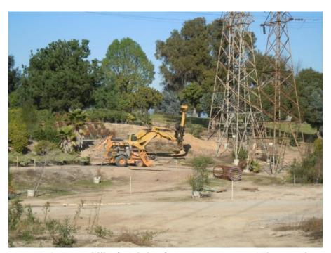
**Figure 4:** Crews drill a foundation for a TSP, Segment 7 66 kV near the Mesa Substation.
