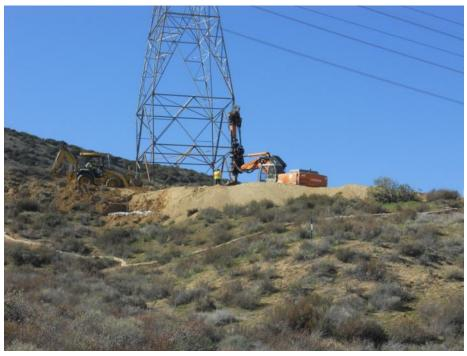
Figure 1: Woodward Brothers drilling foundation for Tower 17, Segment 5.
