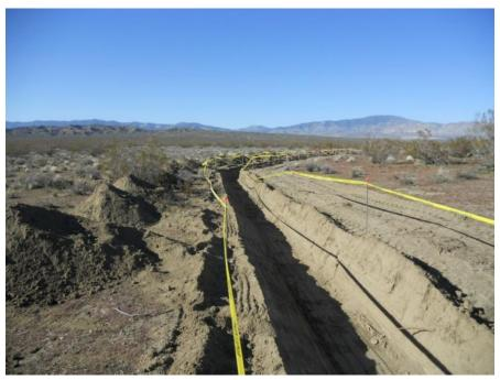
Figure 2: Tortoise fence trench along perimeter of Whirlwind Substation, Segment 9.
