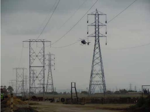
**Figure 7:** A helicopter pulls a sockline for conductor stringing along the Chino–Mira Loma No. 1 line, Segment 8, Phase 2.
