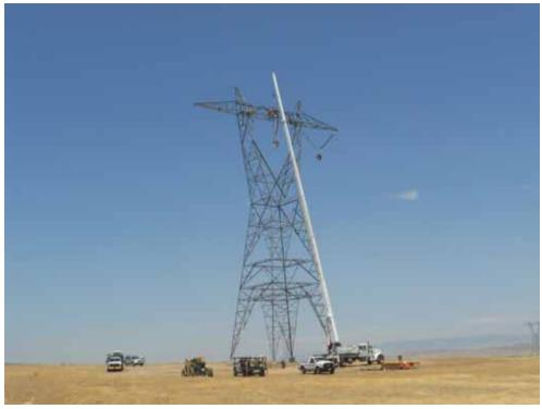
**Figure 3:** H&M wire crew installing travelers on Tower 49 in preparation for wire stringing, Segment 4.
