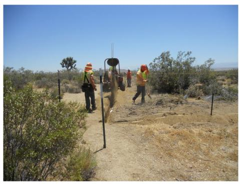
**Figure 2:** Moore Fence crew installing permanent tortoise fencing at Tower 52, Segment 10.
