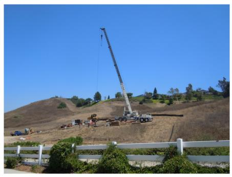
**Figure 5:** Tri-State drills a foundation for an LST in Chino Hills, Segment 8, Phase 1.
