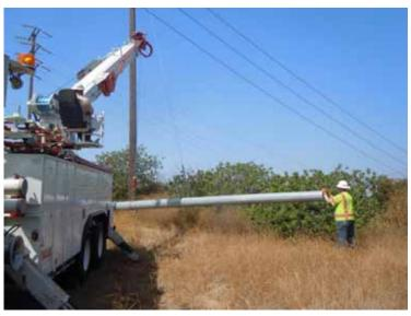
**Figure 5:** An SCE crew erects a lightweight steel pole, Segment 7.
