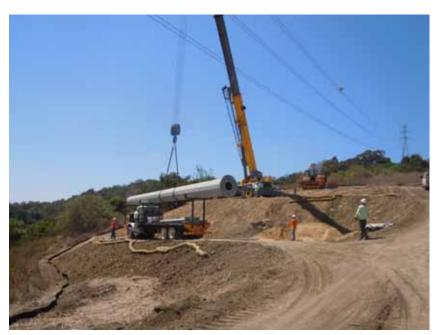
**Figure 8:** A Wilson crew sets an emergency steel pole, Segment 8, Phase 4.
