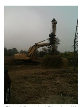
**Figure 6:** Foundation drilling of a 66 kV footing within Whittier Narrows.
