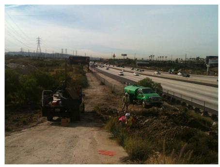
**Figure 5:** Foundation excavation of a 66 kV footing adjacent to the I-605 freeway.
