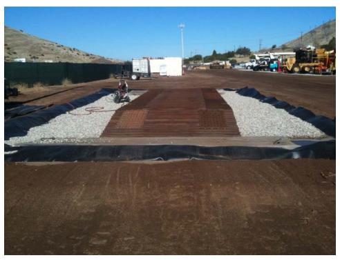
Figure 4: Wash station in the PAR Vincent North Material Yard, Segment 6.
