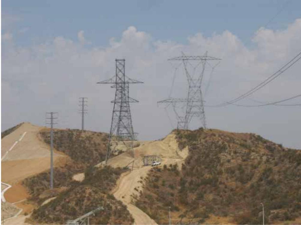
**Figure 1:** Between the Pardee Substation and the beginning of the Shoofly, the new 500 kV towers are being constructed in the center position of an existing SCE right-of-way. The towers on the right are currently supporting the Santa Clara–Vincent line, these towers will be dismantled and the conductor strung onto one side of the new double circuit towers.
