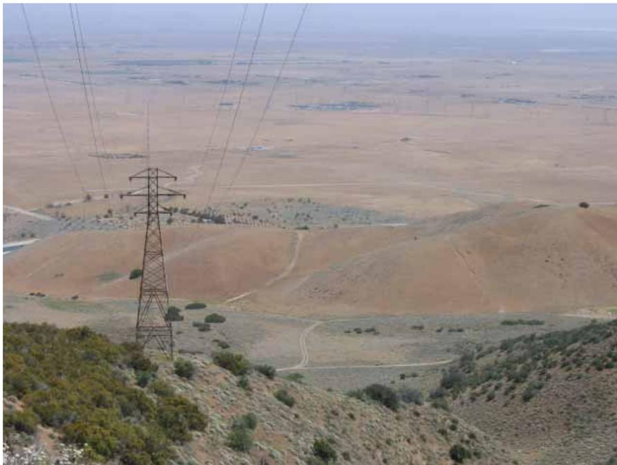
**Figure 2:** In Section 3, the 66 kV towers (seen looking toward the Antelope Valley) will be dismantled in order to construct the new 500 kV Antelope Pardee towers. One side of the lines supported by the 66 kV towers will be relocated to wood poles, the Hughes Lake 12 kV portion of the Project.
