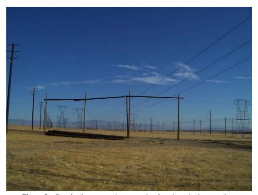
**Figure 3:** Guard pole structure in preparation for wire stringing near the Antelope Substation, Segment 2.
