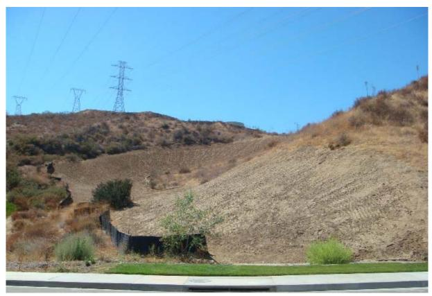
Figure 1: Recontouring of temporary access road along Rock Canyon Road, Section 1.
