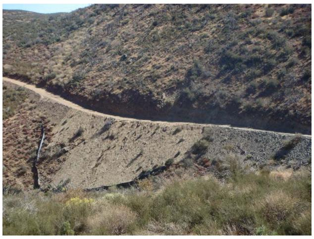
**Figure 2:** Side cast material along access road near Tower 48, Segment 2.
