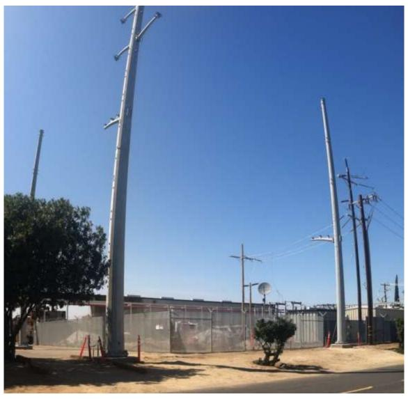
Figure 4 – Three TSPs and a VSAT dish were installed at the Gallo Substation during the subject period. View northwest, 04/15/15.
