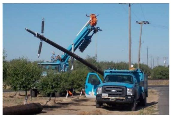
Figure 5 – Crews installed poles along Mercedes Avenue during the subject period. View west (photograph provided by PG&E).
