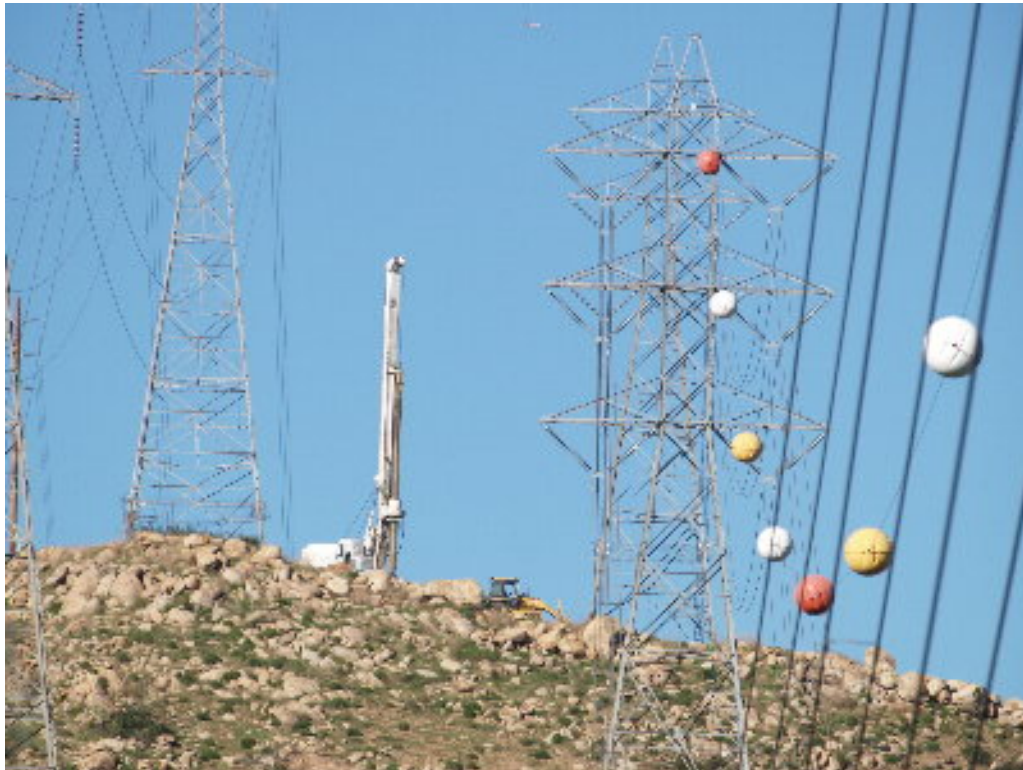
Figure 6 – The drilling at Tower Site 881 was completed during the week.
