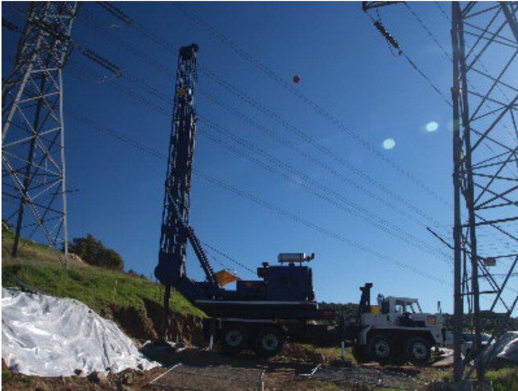
Figure 7 – The drilling continued south of Highway 8.
