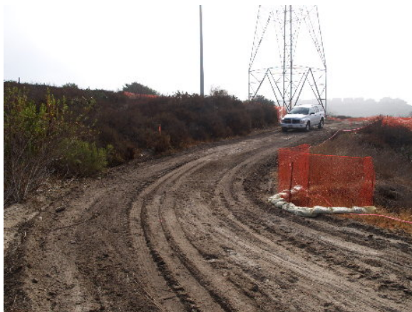
Figure 3-3. The access road between the southern 220 kV tower and the Viejo Substation was eroding due to natural drainage. Steel plates, and later rock, were placed to allow safe passage, October 5, 2004
