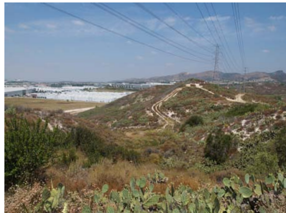
Figure 4-1. Native vegetation on 66 kV right-of-way prior to construction, May 2005
