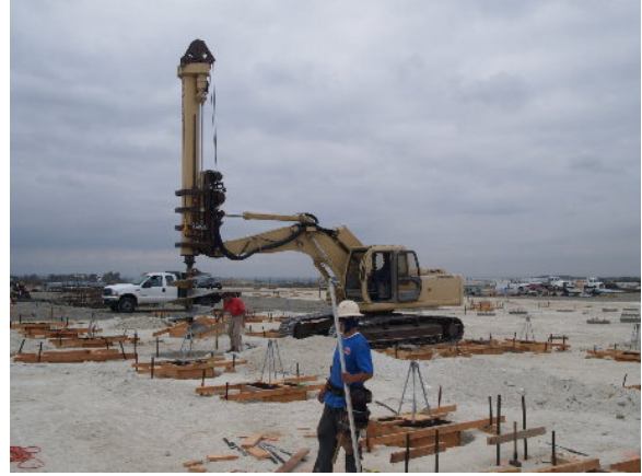
Figure 2-4. Boring machine excavating foundations for supports in the Viejo Substation, September 30, 2004
