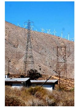
removal of 116 transmission towers (average height 83 feet for single-circuit towers and 141 feet for double-circuit towers) and installation of 93 new towers (average height 157 feet). The new towers would interconnect at the Devers Substation.
