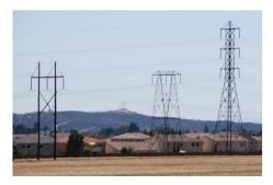
Project work in this segment would require removal and replacement of three existing 220 kV transmission lines. This includes removal of 175 towers (average height 90 feet for single circuit towers and 139 feet for double circuit towers) and installation of 136 new towers (average height 142 feet).
