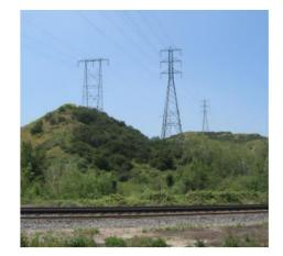
Segment 3 includes three separate sets of existing towers that would be removed and replaced with two sets of new 220 kV double circuit towers. Project work within Segment 3 would include removal of 116 towers (average height 86 feet for single-circuit towers and 139 feet for double-circuit towers) and Installation of 133 towers (average height 143 feet).
