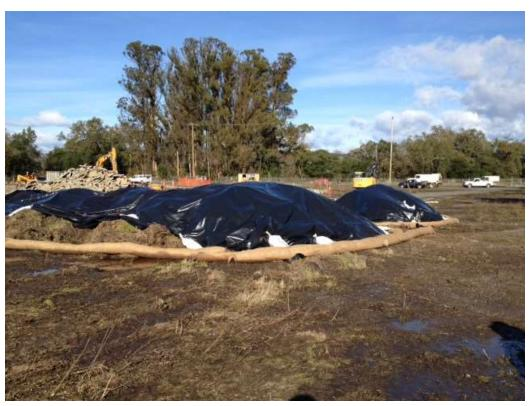
Figure 2 – Substation site vegetation grubbed and graded with stockpiles covered in plastic and surrounded with straw wattles, November 28, 2016.
