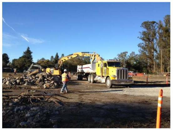
Figure 4 – Demolished concrete and debris being loaded into haul truck at substation site, December 1, 2016.
