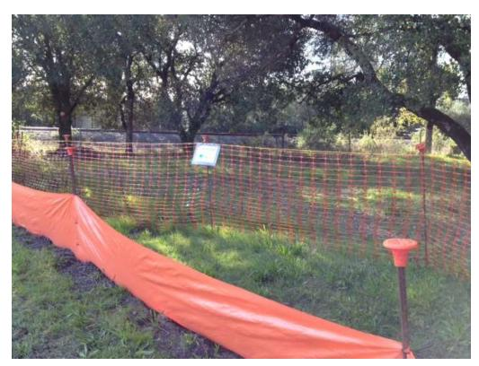
Figure 1 – Silt fence and ESA fencing installed at substation site, November 28, 2016.
