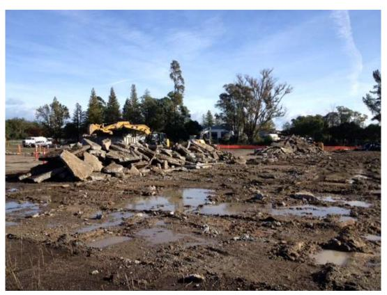
Figure 3 – Demolition of existing concrete pads at substation site, November 28, 2016.
