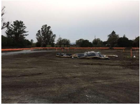
Figure 1 – Substation site with stockpiles covered with plastic and surrounded by fiber rolls, December 7, 2016.
