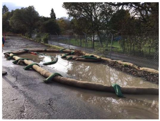
Figure 4 – Drainage inlets with BMPs installed on north side of substation site, December 9, 2016.
