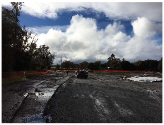
Figure 3 – Demolition of existing concrete pads at substation site, December 9, 2016.
