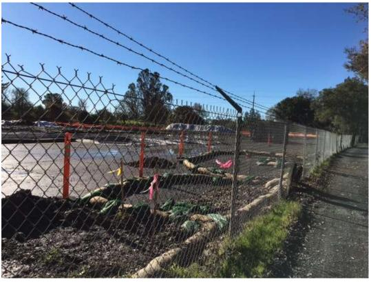
Figure 6 – Drainage inlets on the north side of the substation site after storm event, December 16, 2016.
