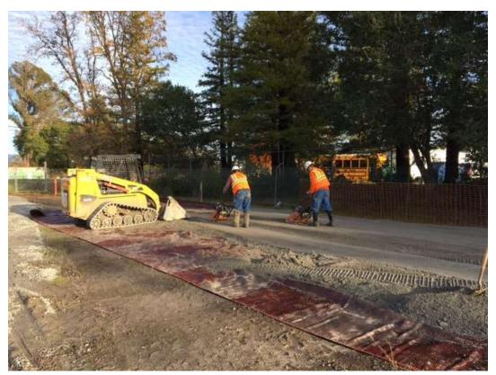
Figure 2 – Compacting base rock on southern side of substation site, December 12, 2016.
