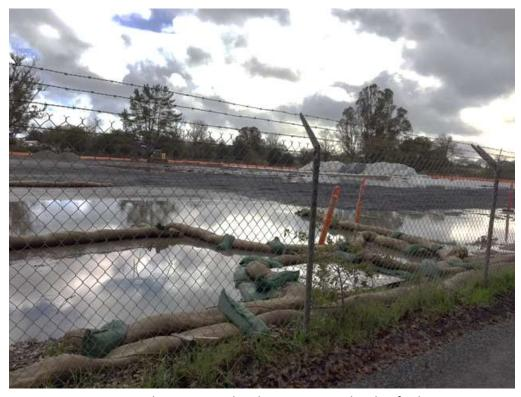
Figure 2 – Drainage inlets protected with BMPs on north side of substation site – view southwest, January 20, 2017.
