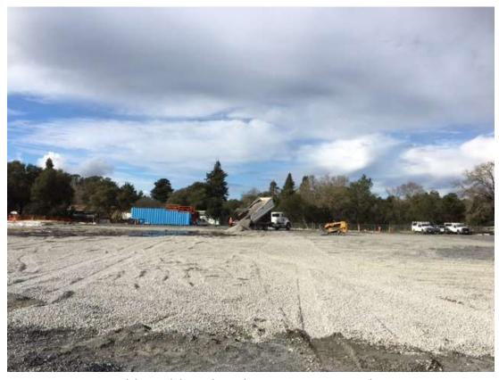
Figure 4 – Base rock being delivered to substation site – view north, January 25, 2017.
