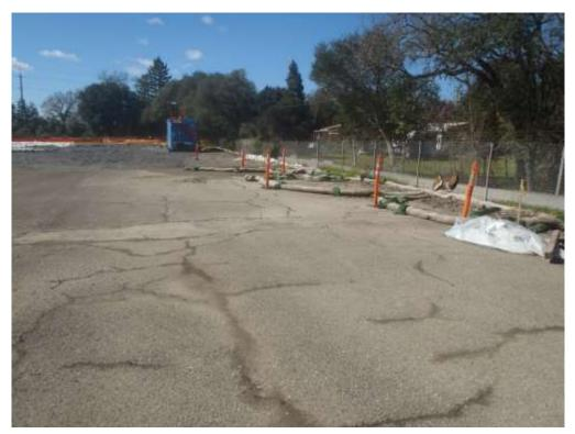
Figure 2 – Drainage inlets protected with BMPs on north side of substation site – view west, February 27, 2017. Photo courtesy of PG&E.
