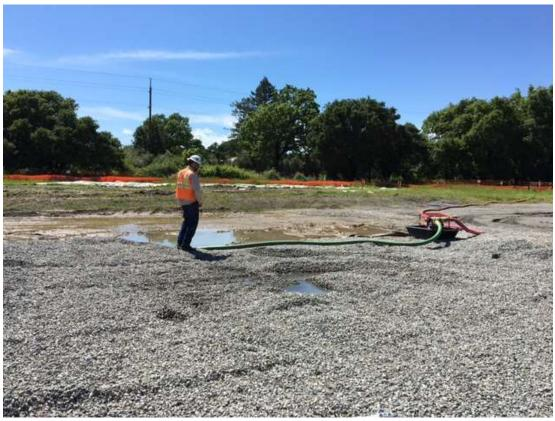
Figure 3 – Crews pumping water at substation site – view northwest, April 20, 2017.
