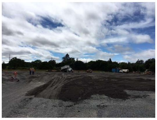
Figure 1 – Base rock being delivered, spread, and compacted at substation site – view northwest, April 26, 2017.
