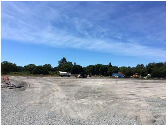
Figure 4 – Spreading and compacting base rock at substation site – view northwest, April 28, 2017.
