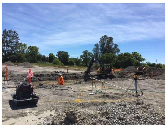
Figure 5 - Excavating for switchgear foundation at substation site - view southwest, April 28, 2017.
