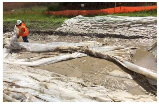
Figure 2 – Removing plastic lining from stormwater ponds at substation site – view southwest, April 26, 2017.
