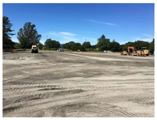
Figure 2 – Spreading and compacting base rock at substation site – view west, May 4, 2017.
