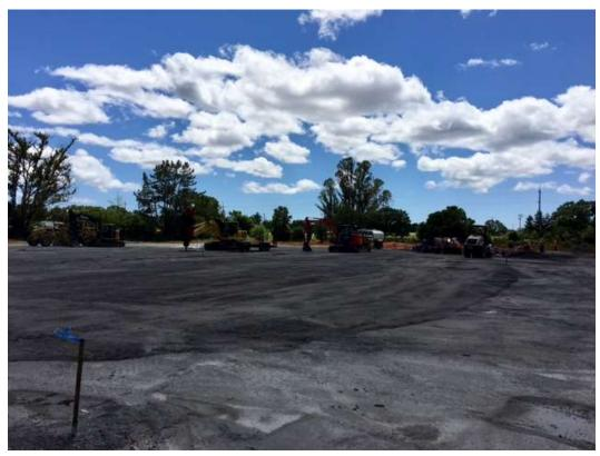
Figure 3 – Spreading and compacting additional base rock for pad at substation site – view west, May 12, 2017.
