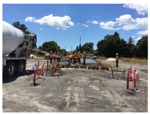
Figure 2 – Pouring cement for switchgear foundation at the substation site – view west, May 15, 2017.
