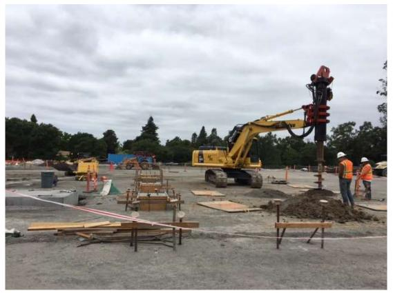
Figure 3 – Drilling pier holes on south side of substation site – view north, May 26, 2017.
