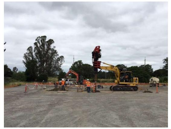
Figure 2 – Drilling pier holes on south side of substation site – view west, May 26, 2017.
