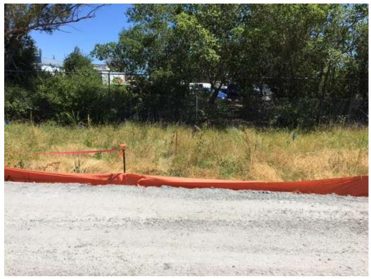
Figure 3 – Silt fence torn and pushed down on south side of substation site – view south, May 31, 2017.
