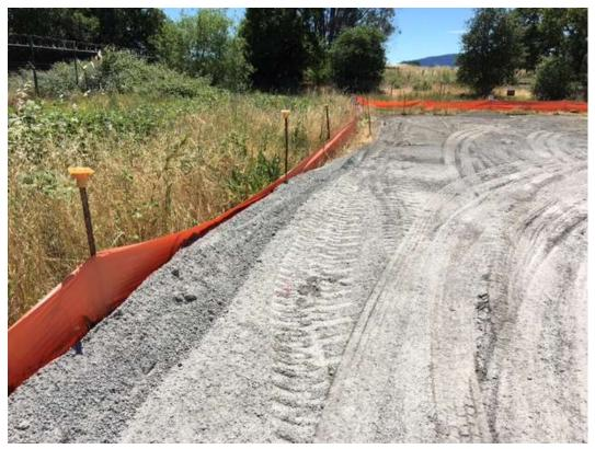
Figure 4 – Base rock pushed up against silt fence on south side of substation site – view west, May 31, 2017.
