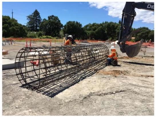
Figure 2 – Rebar work for pier foundations on south side of substation site – view northwest, May 31, 2017.
