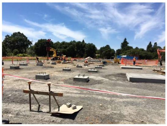
Figure 4 – Foundation work on the southwest side of substation site – view north, June 5, 2017.
