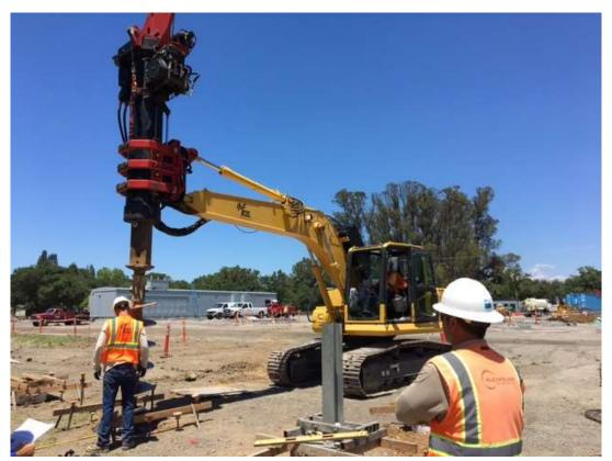
Figure 4 – Drilling for perimeter fence on west side of substation site – view northeast, June 13, 2017.
