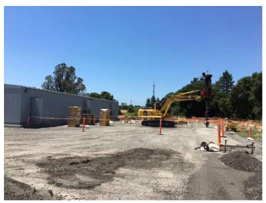
Figure 2 – Drilling foundation holes for perimeter fence on north side of substation – view west, June 20, 2017.
