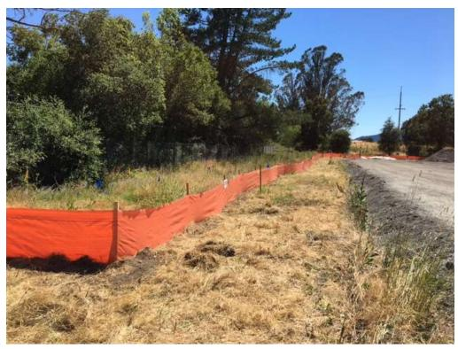
Figure 3 – Relocation of silt fence on south side of substation site – view west, June 26, 2017.
