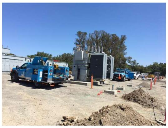
Figure 2 – Welding transformer to foundation pad – view east-northeast, July 12, 2017.
