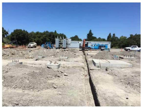
Figure 4 – Foundation and grounding work – view north, July 12, 2017.
