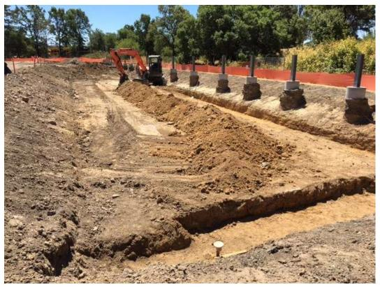
Figure 1 – Excavation of SPCC pond on west side of substation – view south, July 21, 2017.
