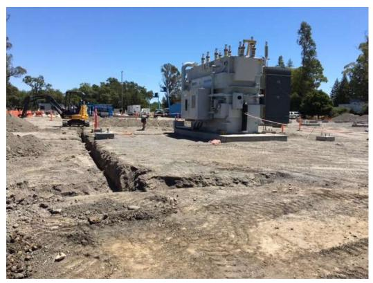
Figure 2 – Grounding work and excavations at the transformer – view east, July 21, 2017.
