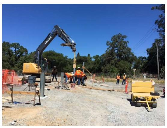
Figure 3 – Drilling pier holes for perimeter wall foundations on east side of site – view north, July 21, 2017.
