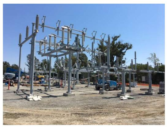
Figure 4 – Installation of switches and insulators on dead-end structures – view southeast, August 18, 2017.
