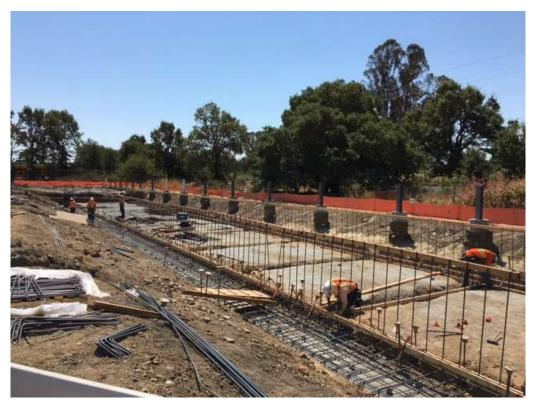
Figure 1 – Tying rebar in the SPCC ponds on west side of site – view southwest, August 18, 2017.
