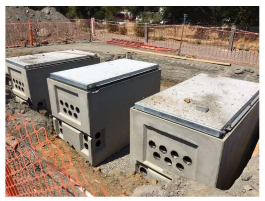
Figure 3 – Last two pull boxes set on northern perimeter – view northwest, August 18, 2017.
