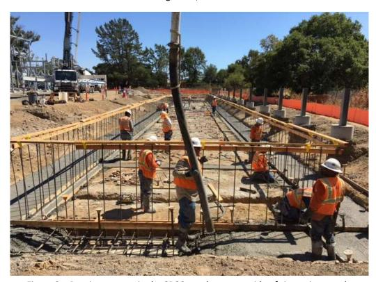
Figure 2 – Pouring cement in the SPCC ponds on west side of site – view south, August 30, 2017.
