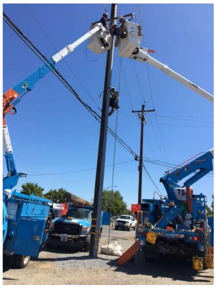
Figure 5 – Crews working on 12 kV riser cable jumper at Pole b4 – view southeast, August 30, 2017.
