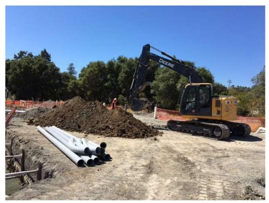
Figure 3 - Excavating trenches for conduit to pull boxes set on northern perimeter – view northwest, August 30, 2017.
