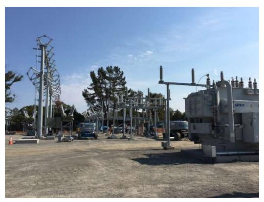
Figure 3 – Installing switches and insulators on dead-end structures – view south, September 6, 2017.
