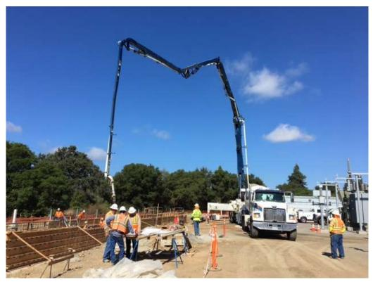
Figure 2 – Pouring cement slurry in wall panel forms in the SPCC ponds – view north, September 14, 2017.
