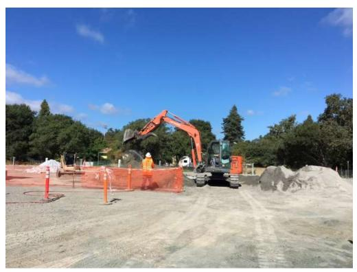
Figure 1 – Backfilling conduit trenches – view north, September 14, 2017.
