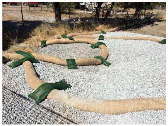
Figure 4 – Additional BMPs installed around drainage inlet – view northeast, September 21, 2017.
