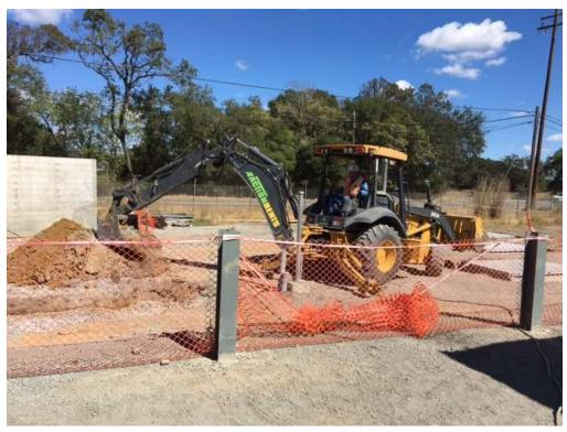
Figure 1 – Excavating conduit trenches and pull boxes – view east, September 21, 2017.
