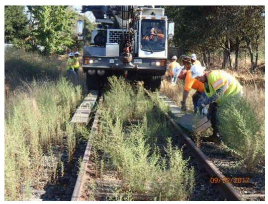
Figure 5 – Crane driving across planks atop the railroad tracks – view south, September 25, 2017. Photo courtesy of PG&E.
