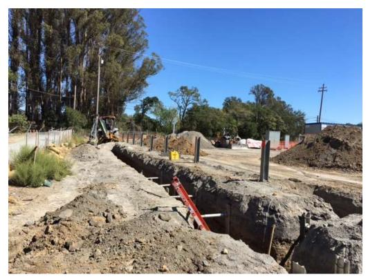
Figure 1 – Excavating conduit trenches along substation northern perimeter – view east, September 27, 2017.
