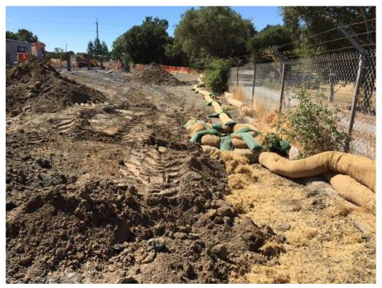
Figure 3 – Soil pushed up against drainage inlet on northern perimeter – view west, September 27, 2017.
