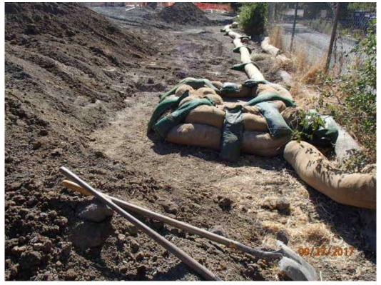
Figure 4 – Soil pulled back from drainage inlet – view west, September 28, 2017. Photo courtesy of PG&E.
