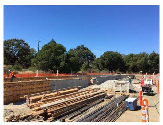
Figure 2 – Installing rebar and wall forms for the SPCC pond – view northwest, September 27, 2017.
