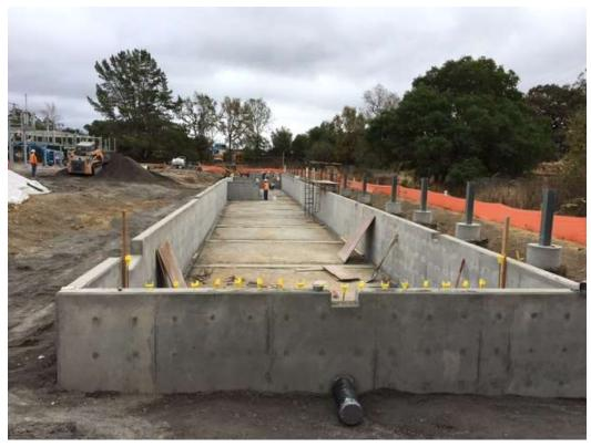
Figure 3 - Backfilling and compacting fill around SPCC pond - view south, October 19, 2017.
