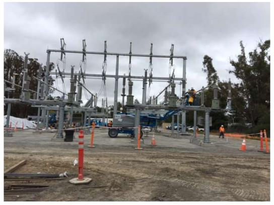
Figure 4 – Installing switches and insulators on dead-end structures – view east, October 19, 2017.
