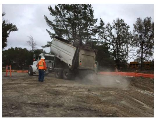
Figure 2 – Delivery of base rock and sand – view south, October 19, 2017.
