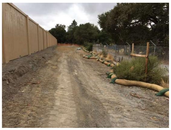
Figure 5 – Additional BMPs installed along northern perimeter and around drainage inlets – view west, October 19, 2017.
