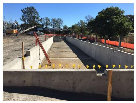
Figure 2 – Backfilling and compacting around SPCC pond – view south, October 27, 2017.
