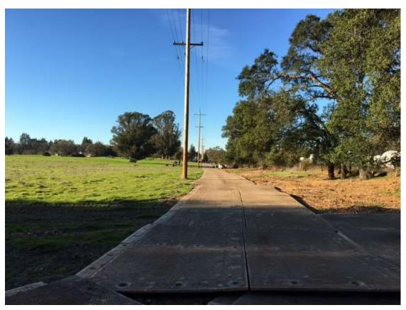
Figure 5 – Matting for equipment and vehicles to drive on to TSP location in field west of substation site - view north, December 6, 2017.
