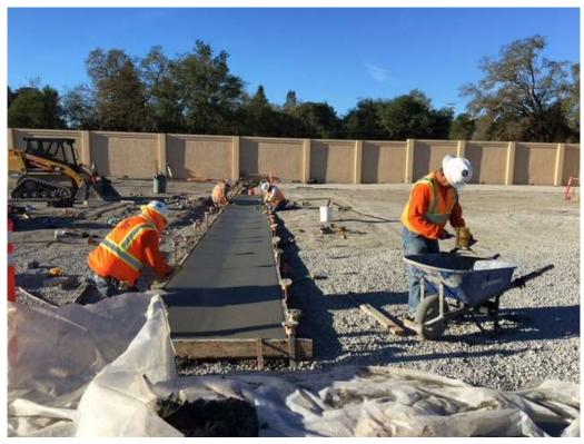
Figure 2 – Forming cement V-ditches on the north side of the substation – view north, December 6, 2017.
