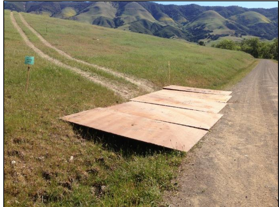
Example of an existing unpaved access road, temporary crossing, and overland route
